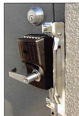
Photo shows a back door lock. The latch guard was modified to fit around the OmniLock
